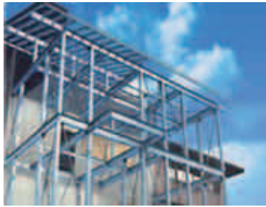
(1) Structural post and beam for residence
